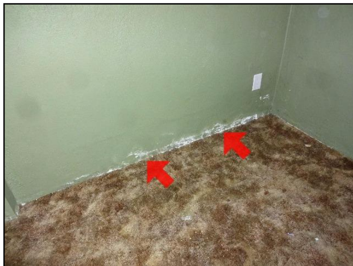
6. Efflorescence
